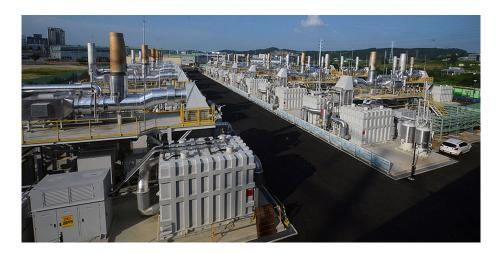
**59 MW power plant based on twenty-one FuelCell Energy 3000 systems** Project developed by POSCO, Korea Hydro Nuclear Power Co. (KHNP) and Samchully Gas Co in South Korea is an example of large systems based on 2.8MW FuelCell Energy 3000 plants.
