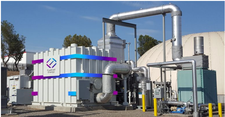
1.4MW carbonate fuel cell
