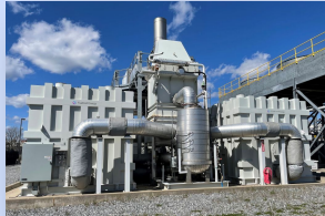
Carbon Recovery 1.3-1.8 MW power 20+ Mt/day CO 2
